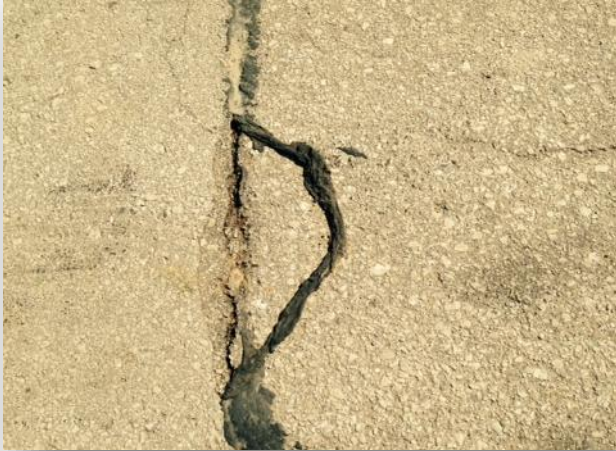
Adhesive Failure
