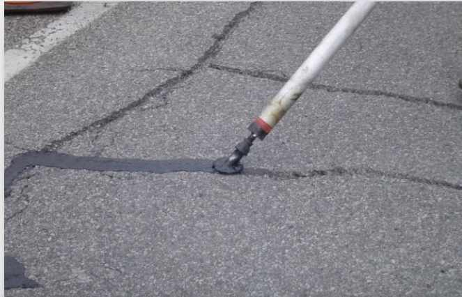
Crack Sealing
