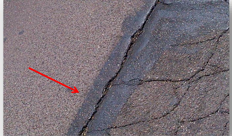
Cohesive Failure
