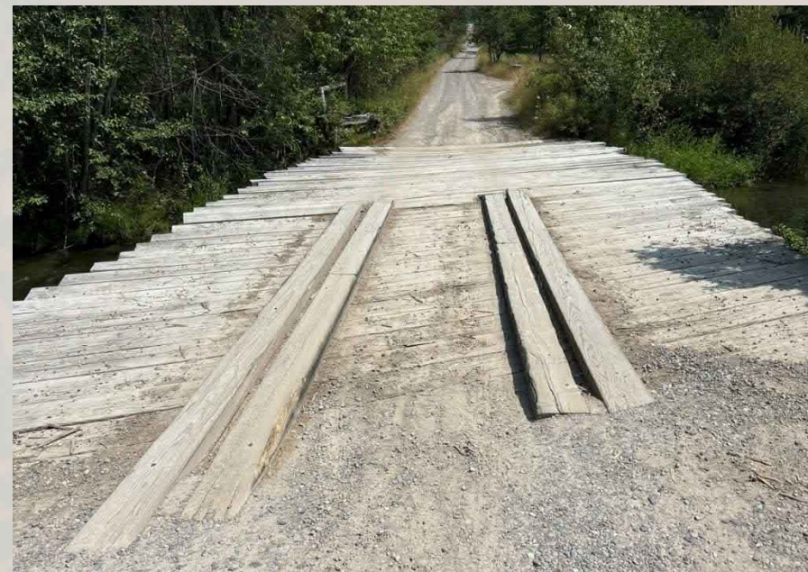
Bridge Centerline and Up Stream
