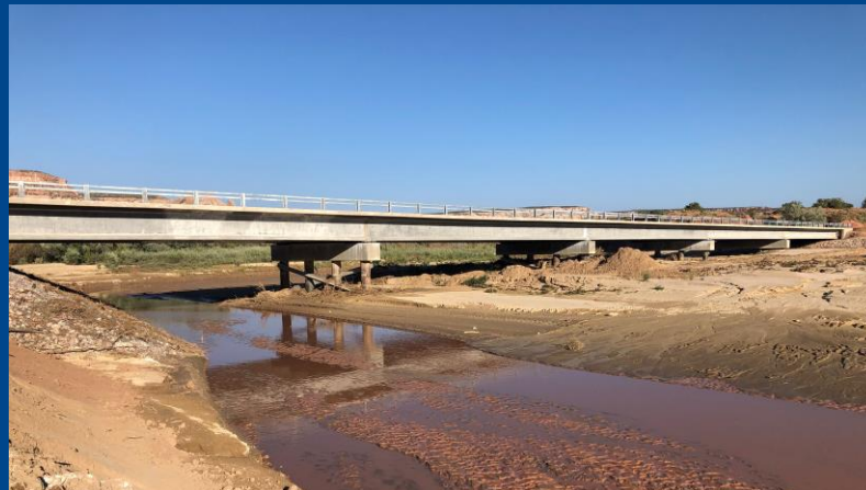
Downstream side of Bridge
