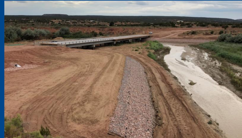
Upstream Wire-tied Riprap Protection
