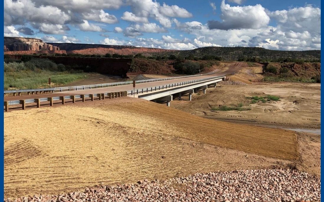
New N9402 5-Span Concrete Bridge in Lupton, AZ
