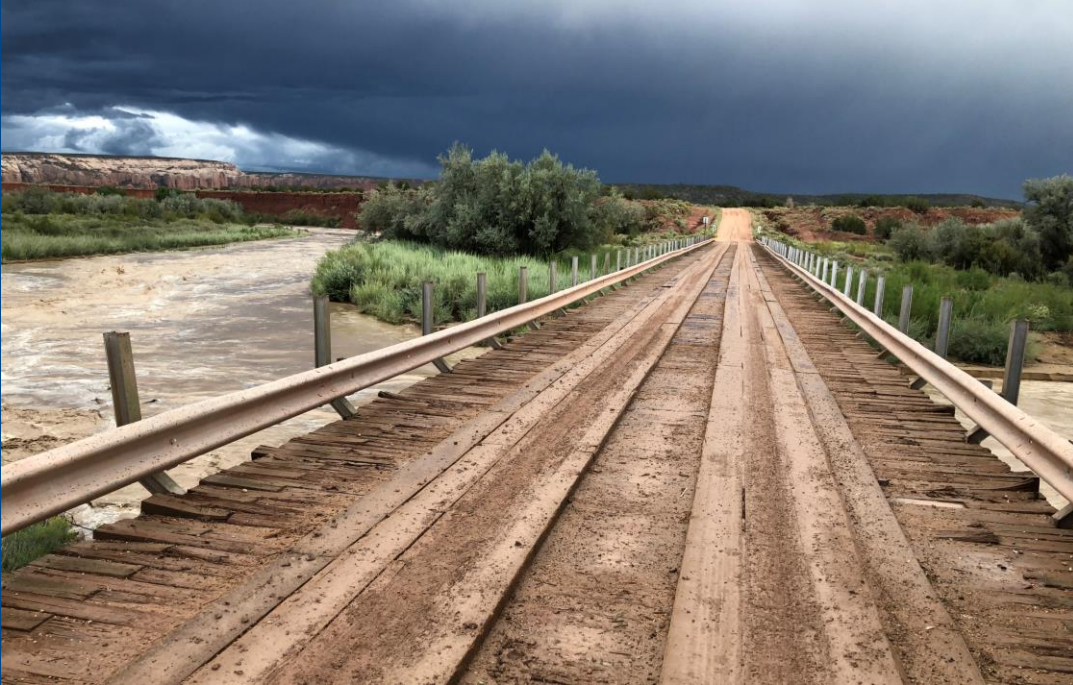
Old N9402 Steel Military Bridge in Lupton, AZ
