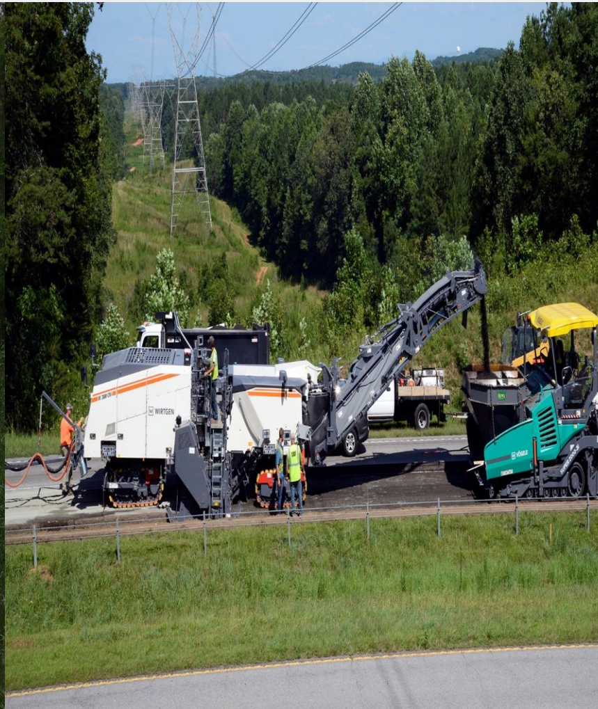
Paver Laid FDR
