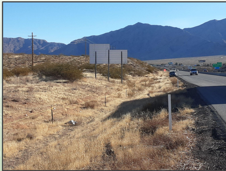
Site protection using t-posts/rope
