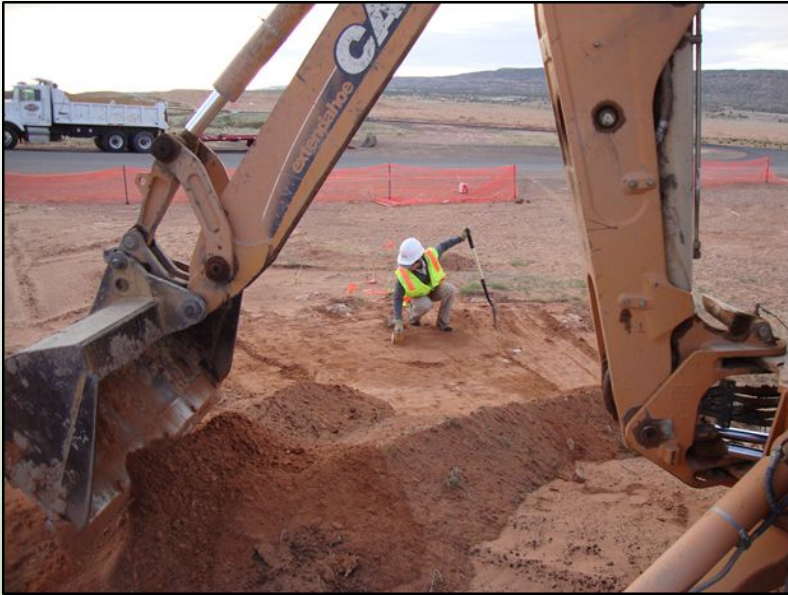
Excavation along US-160
