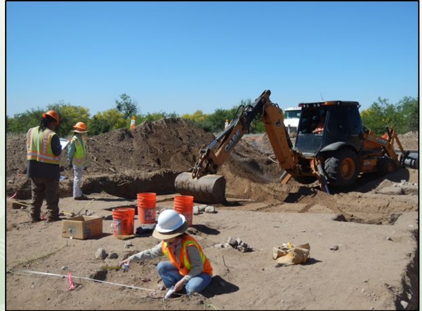
Excavation along SR-86
