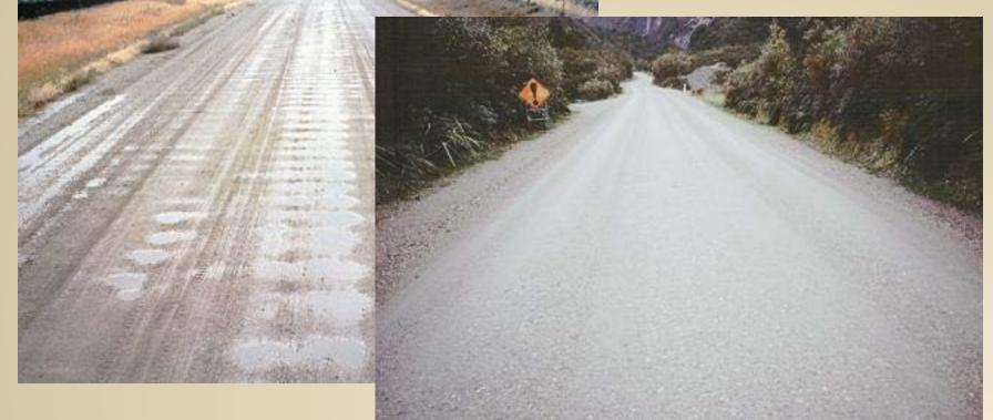
Clear illustration of 2% crown on the road to the left and 4% on the road to the right. Water will not drain off an aggregate surface with only 2% crown. This must be addressed in design and during construction.
