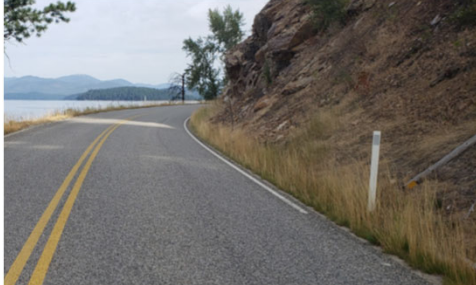
Figure 1. Edge lines and delineators improve visibility on horizontal curves. Source: Matt Mulder, Bonner County, Idaho.
