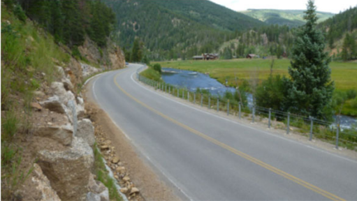
Figure 3. A high-tension cable barrier preserves views of the landscape while shielding vehicles from a steep drop-off. Source: FHWA.
