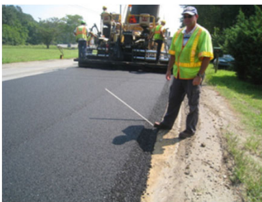
Figure 6. Paving a Delaware roadway with SafetyEdge SM . After paving, a graded shoulder will become flush with top of the pavement, covering the sloped edge. Source: FHWA.
