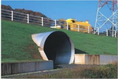
Corrugated Steel Pipe (Buried Steel Bridge)
