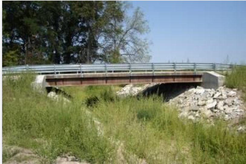
Audrain County, MO Bridge 411
