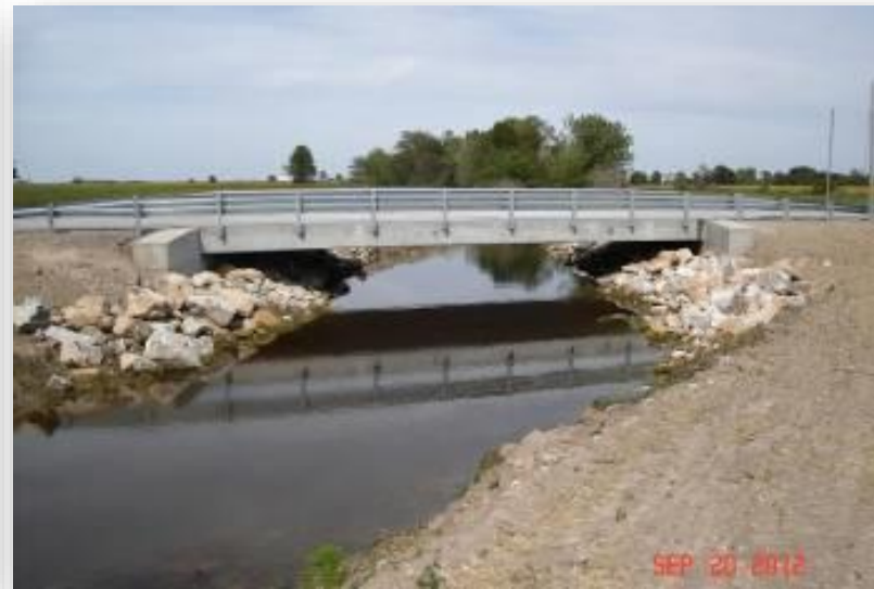
Audrain County, MO Bridge 336
